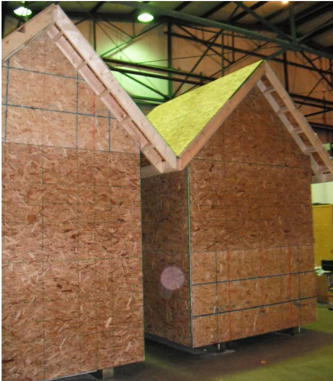
Figure 1 Experimental Test Units during Construction
